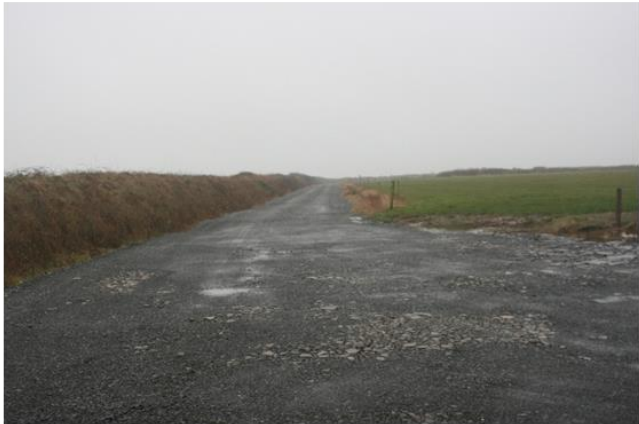
Road Leading to site
