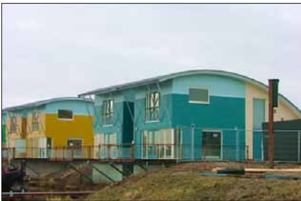
Floating houses built near the water's edge.
