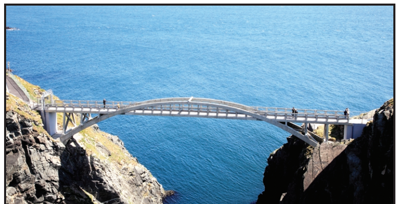
Mizen Head footbridge: almost identical to the original bridge
