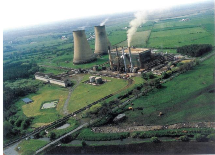
Ferbane Generation Station.
