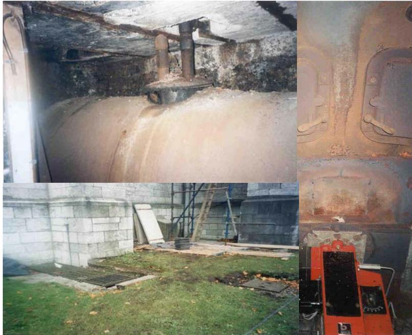
The original heating system consisted of a solid fuel boiler in an underground chamber, which circulated water using gravity circulation through banks of six-inch diameter cast iron pipes. All of these pipes were located in underground ducts and heat was circulated through floor grilles, which were strategically placed around the Cathedral.
