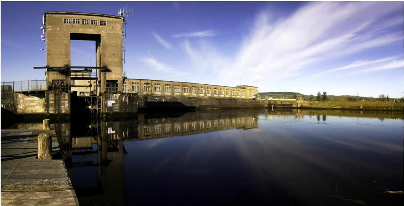
Ardnacrusha hydroelectric power station, Co. Clare
